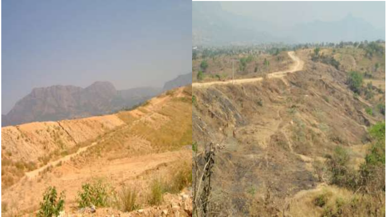
Plate 15: Farin Ruwa Dam Embankment
