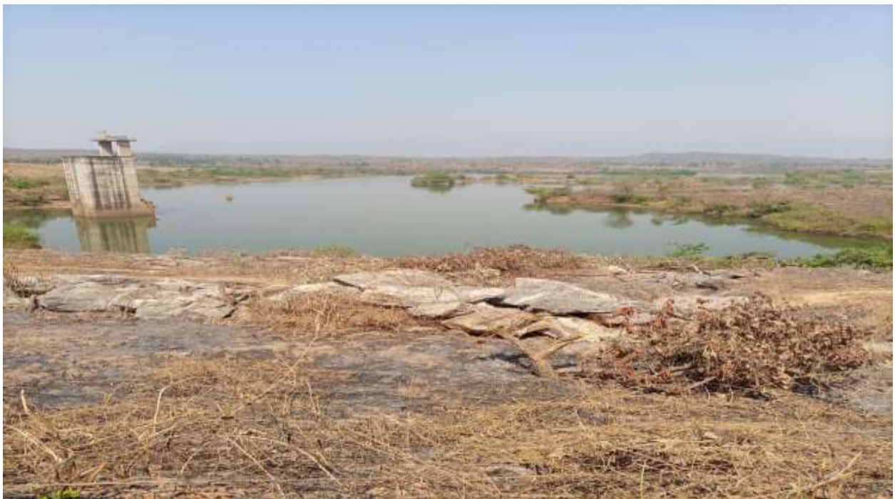
Plate 16: Farin Ruwa Dam Intake Tower
