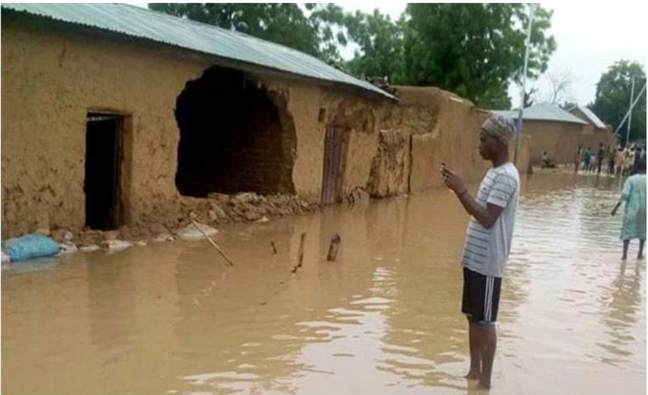
Figure 1.5: Houses destroyed by flood in Jigawa State 2020.
