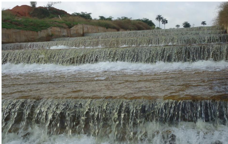
OGWASHI-UKU DAM SPILLWAY
