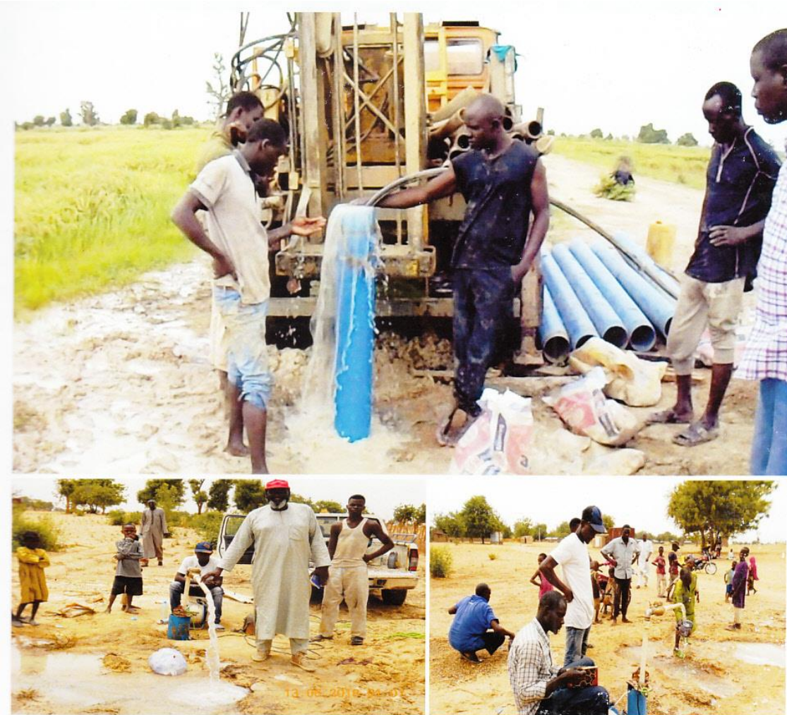
DEEP IRRIGATION BOREHOLES DRILLING AND PUMPING TEST AT UDUBO-WABU DRIP IRRIGATION SCHEME
