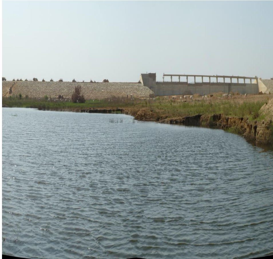
A Section of the Reservoir
