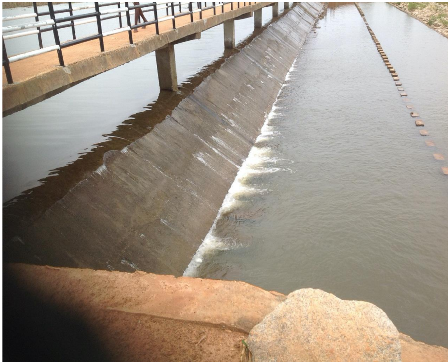
GIMI DAM SPILLWAY
