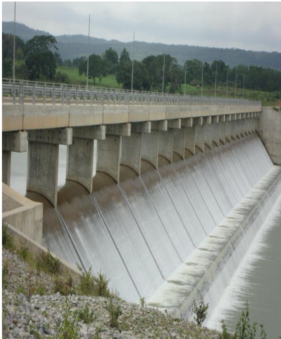
GURARA MULTIPURPOSE DAM
