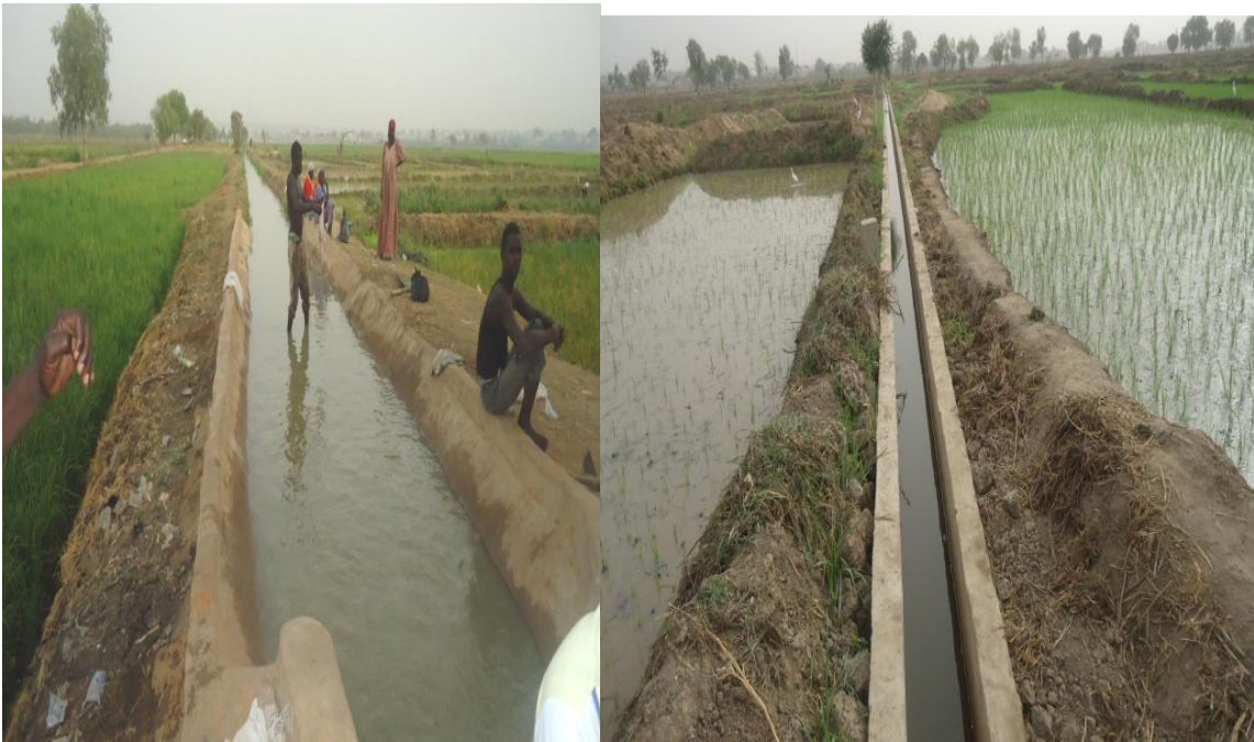
Rehabilitated Primary and Secondary Canals
