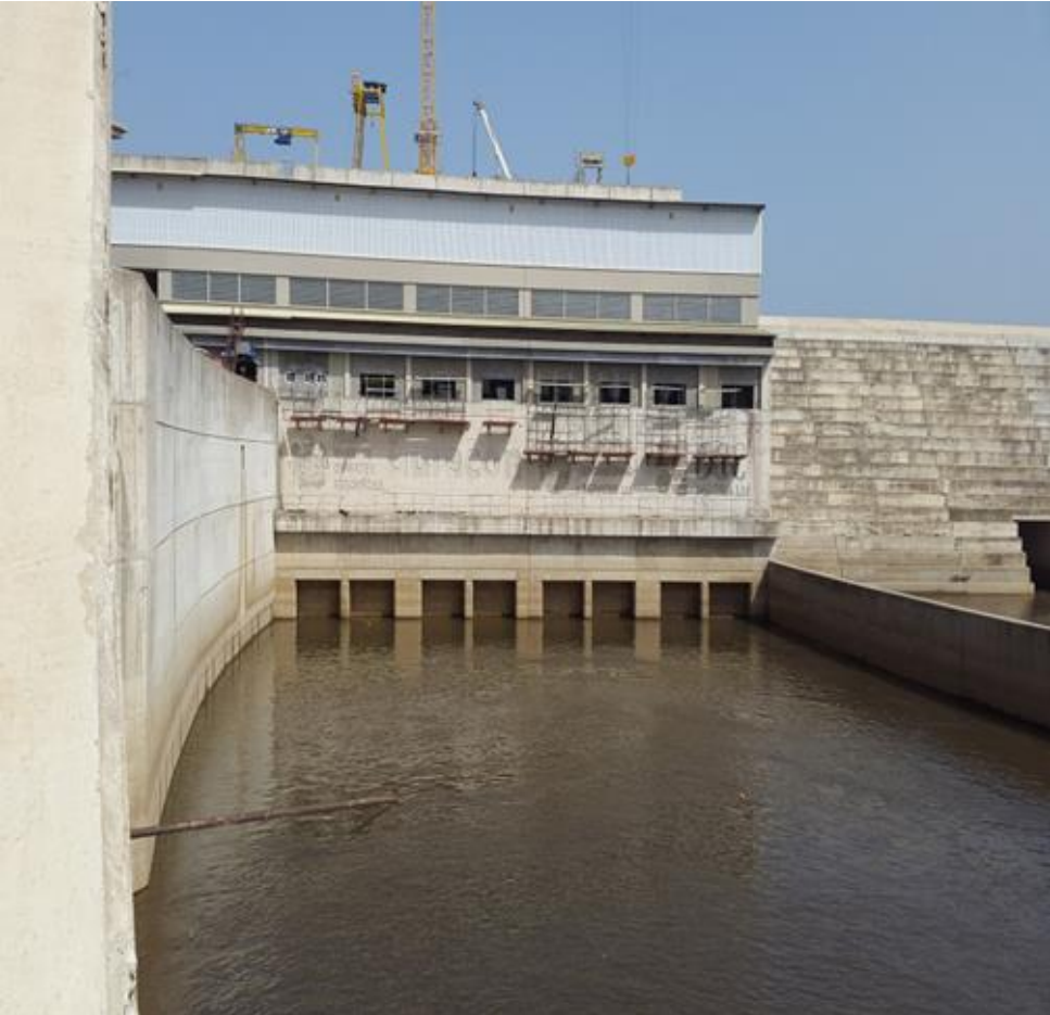
KASHIMBILLA DAM HYDROPOWER PLANT
