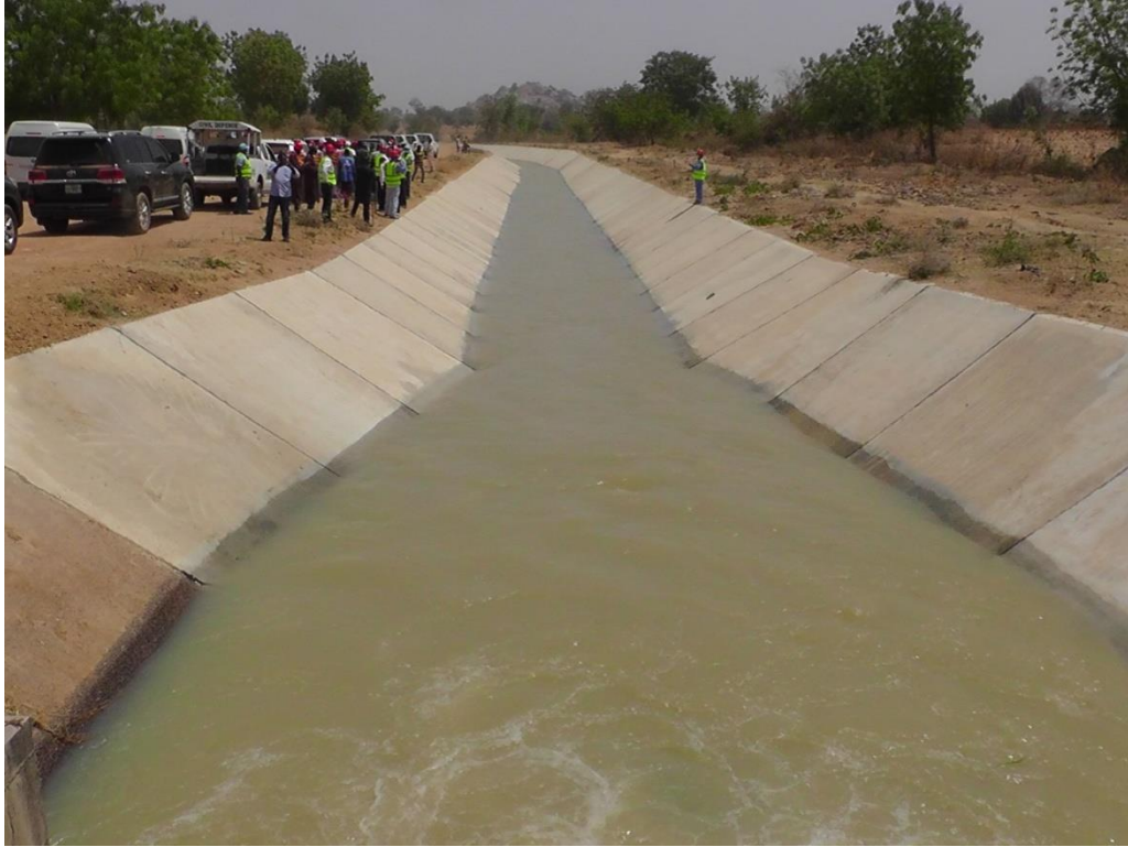
Part of the rehabilitated irrigation structures at Kano River Irrigation Project
