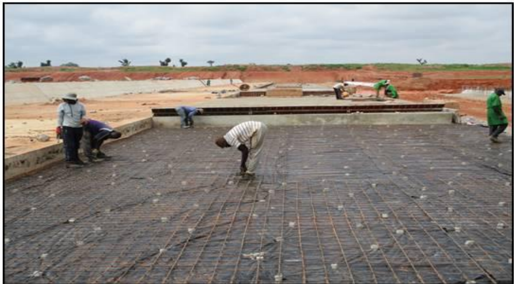
Arrangement and Fixing of Reinforcement bars in Embedded Stone Slab
