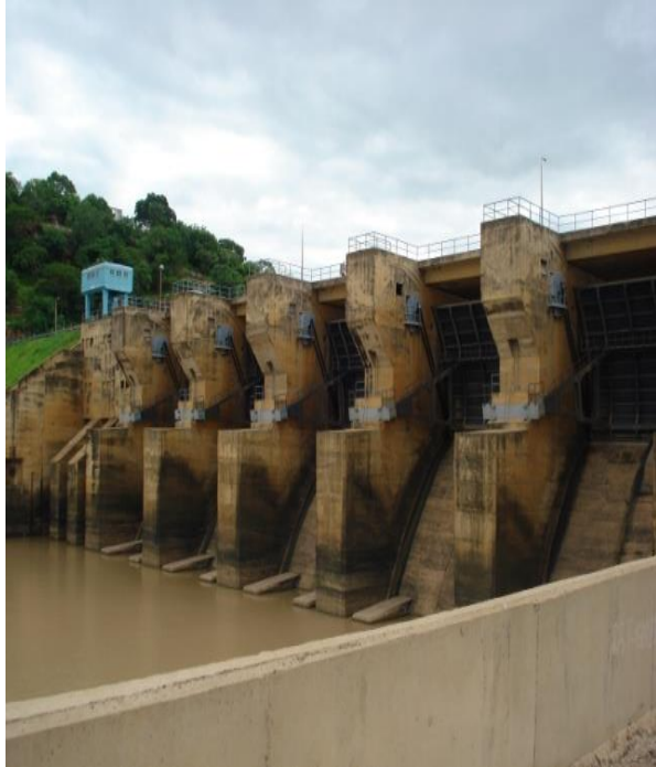
Kiri Dam Reservoir and embankment crest Kiri Dam Spillway Radial Gates & Discharge Channel
