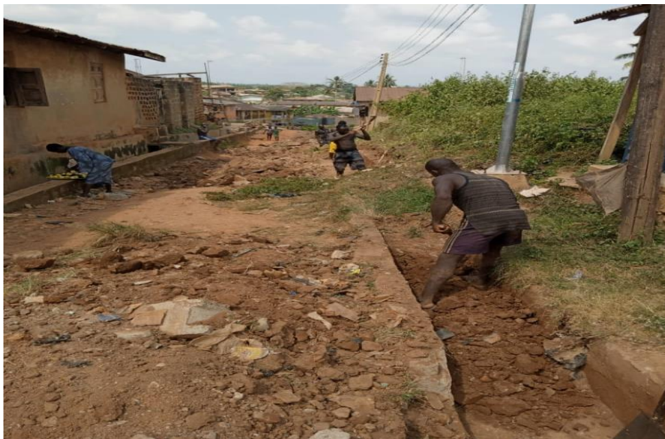
Showing landscape and excavating erosion control Channel
